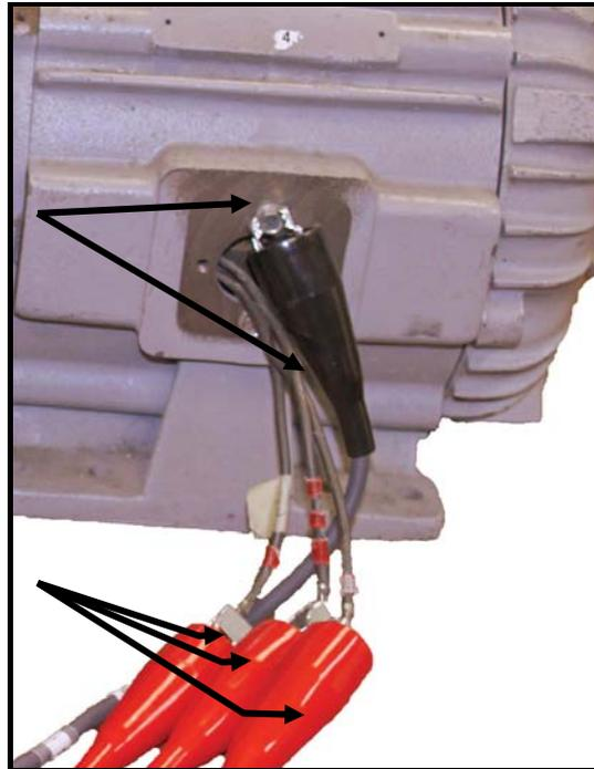
Figure 36. Attach Motor Leads to Test Leads.
