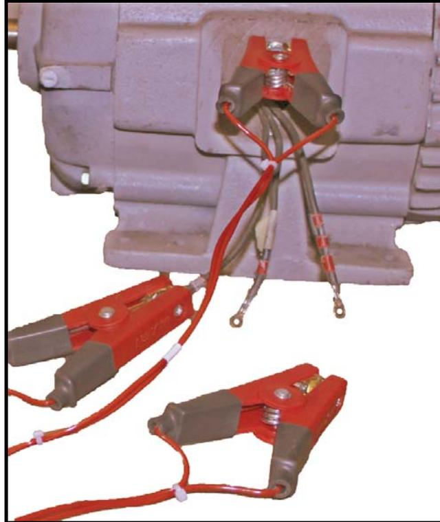
Figure 20. Connect RLC Test Leads to a New Configuration.
